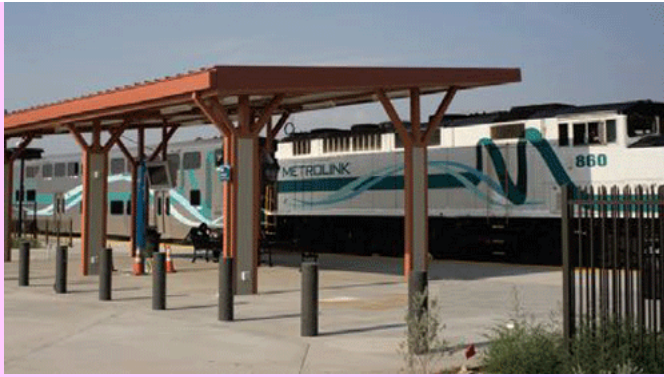
Metrolink Train shown at the Riverside/Hunter Park Station, one of four stations on the Perris Valley Extension!
